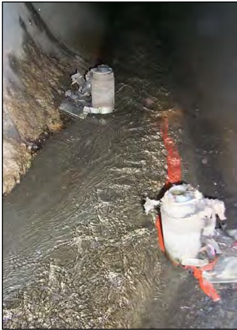
Figure 3: Modified-Norton style trap that has been used by SPU.
