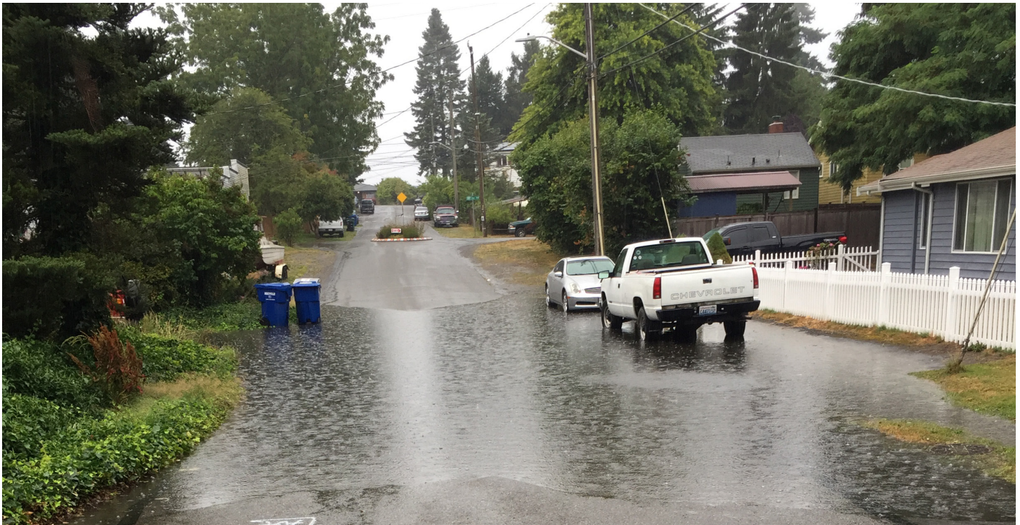
Figure 2.4.E Street flooding across NW 87th St. at 17th Ave NW (Area A on Figure 2.4.D). Upwelling from a drainage inlet is visible behind the white truck; this phenomenon happens multiple times each year.
