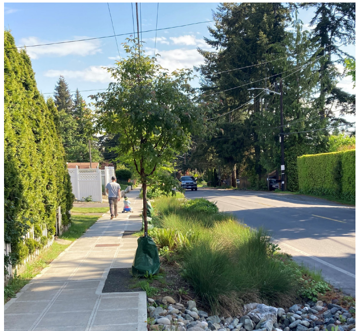
Figure 2.2.D Example sidewalk/bioretention project. In addition to stormwater management, bioretention can improve the pedestrian environment and calm traffic (30th Ave NE Natural Drainage System).
