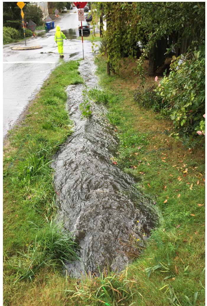
Overflowing ditch and street ponding at the intersection of 17th Ave NW and NW 87th Street.
