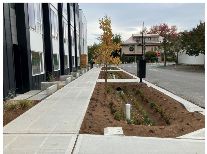
Figure 3.5.2 Queen Mary rowhouse bioretention. A pilot project for “Beyond Code” developer partnering, located just west of the Crown Hill Center.
