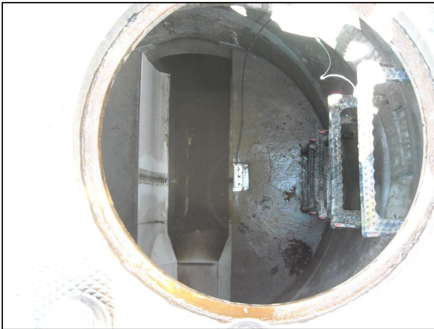
Figure 2.2.2.1b. Photo of R1 Palmer-Bowlus Flume
