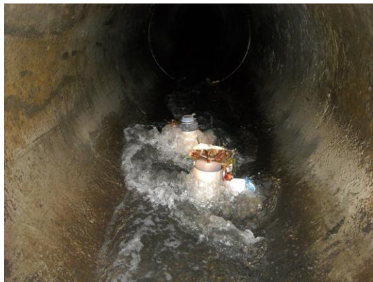
Figure 2.2.2.c. Photograph of C1 Sediment Traps
