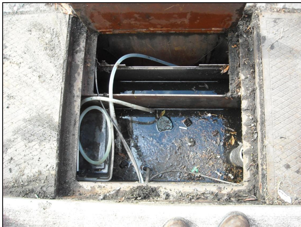
Figure 4.2.2.1f. Inlet Chamber showing Sample Tubing
