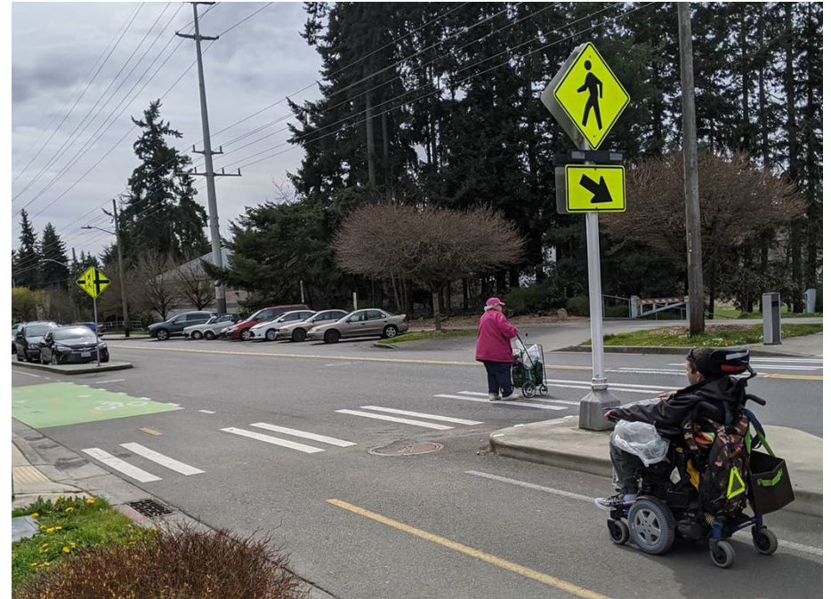
Enhanced pedestrian crossing location and protected bike facility along Linden Ave
