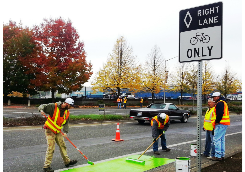
Crews painting a green bicycle lane
