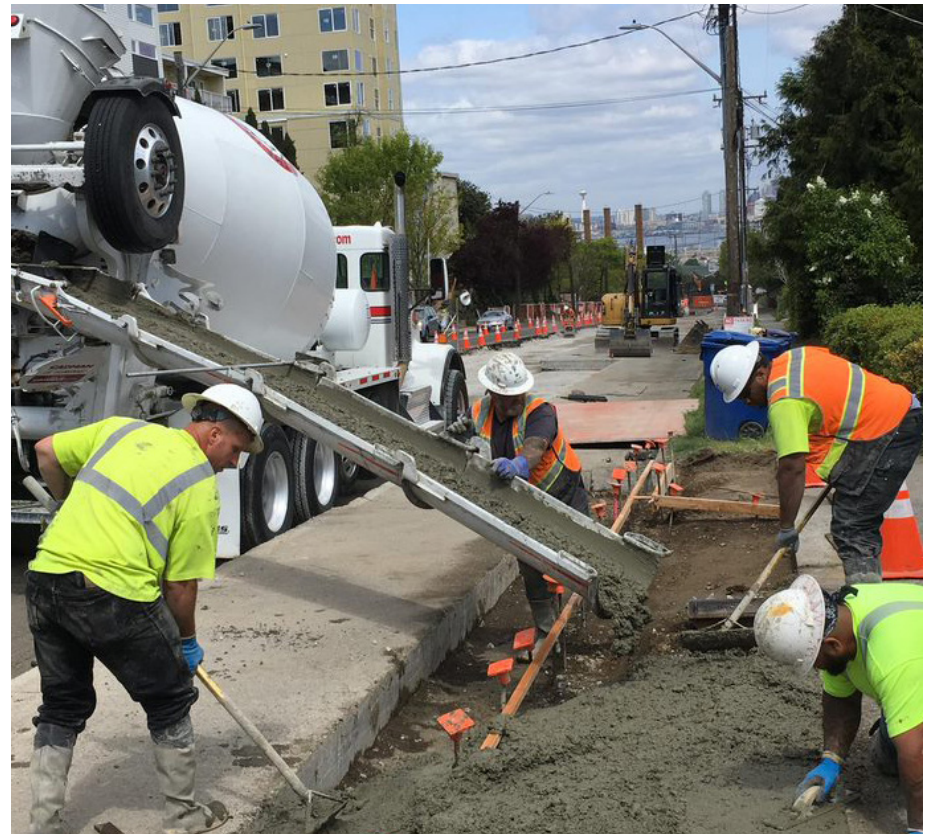
Construction crew at work in West Seattle
