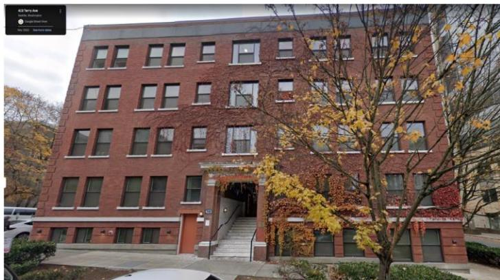
This building was of regular shape, had equal size windows, continuous load paths. The number of window openings can determine the type of upgrades that need to be done inside the building. The building is U shaped and has a smaller floor diaphragm, providing opportunity to build additional lateral support which serves to increase seismic resistance.
