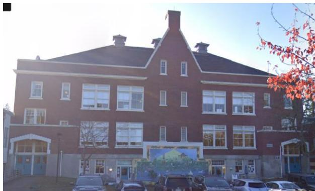
This building is irregular in terms of its shape and window openings. The brick façade will need to be connected to the structural brick behind it. Because this building is a school, and thus a critical structure, additional requirements may be placed because of its use. Additional considerations that may impact seismic considerations include the soil type for liquefaction hazards and foundation elements.
