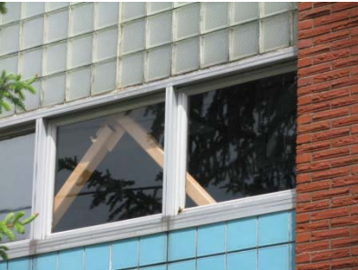
New Building Bracing
