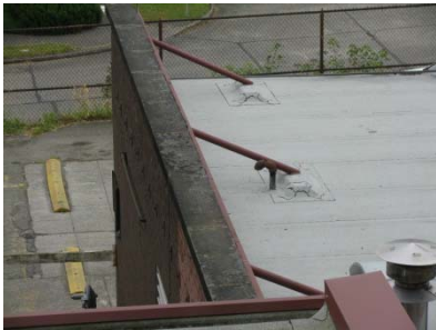
Parapet Bracing
