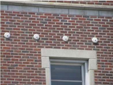
Connecting Floors to Walls
