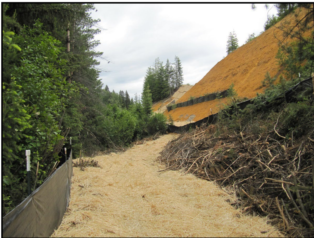
Figure 13. Filter Fence Installed on a Slope.
