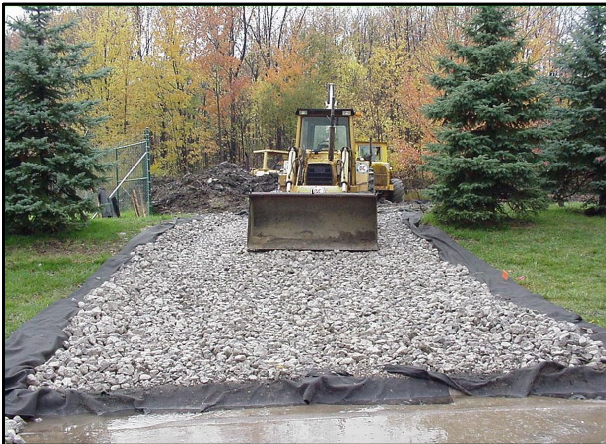
Figure 6. Stabilized Construction Access.
