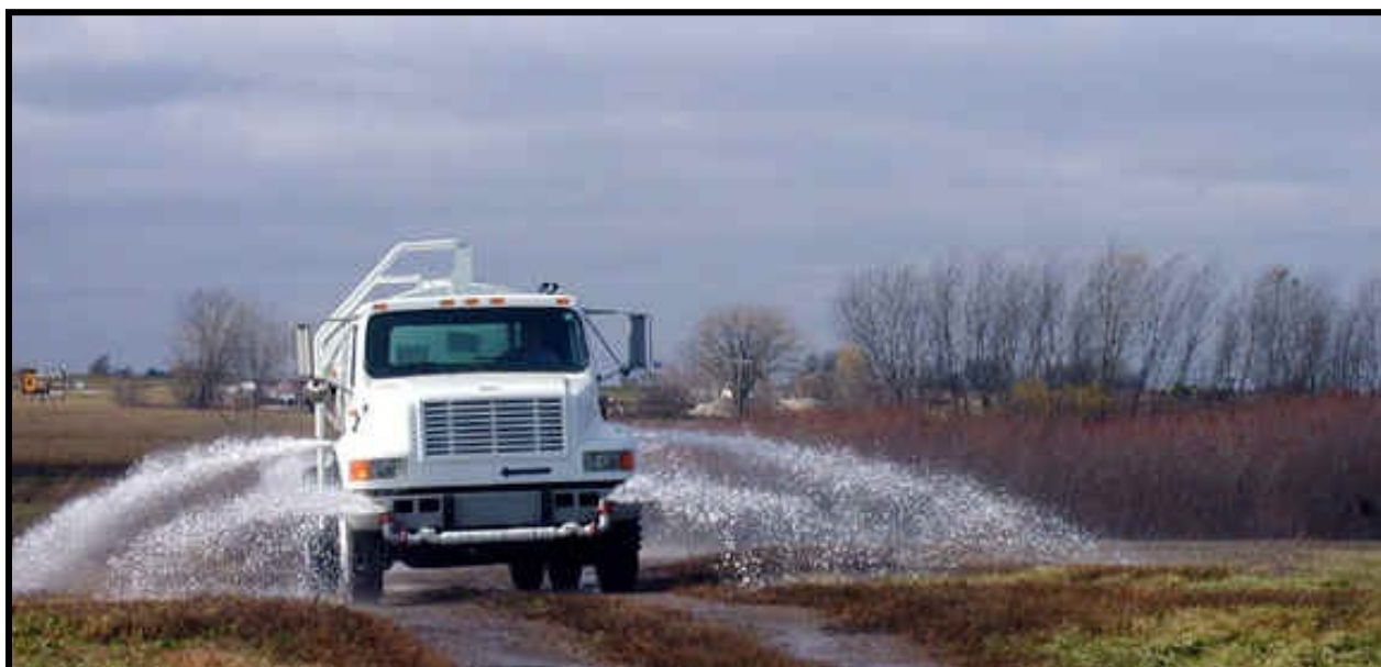
Figure 11. Using a Water Truck for Dust Control.
