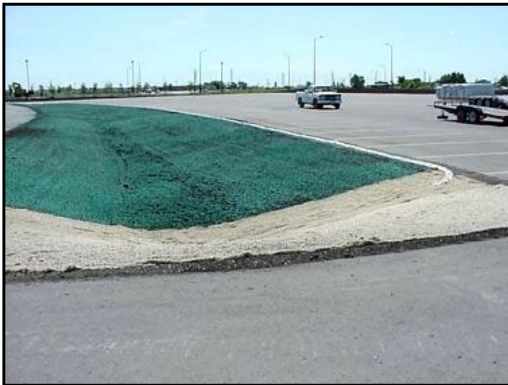
Figure 1. Hydroseeding Method.
