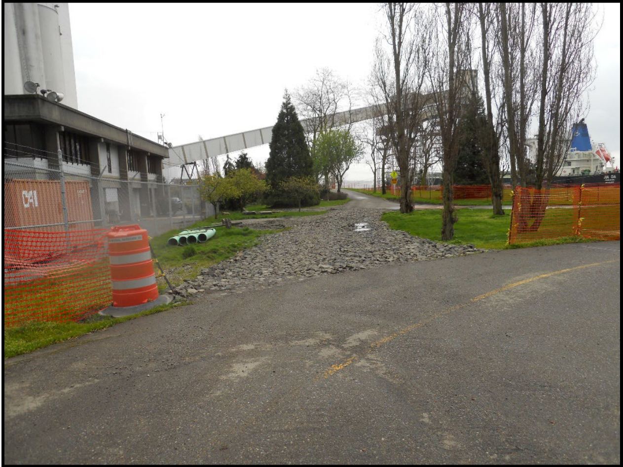
Figure 7. Stabilized Construction Access.
