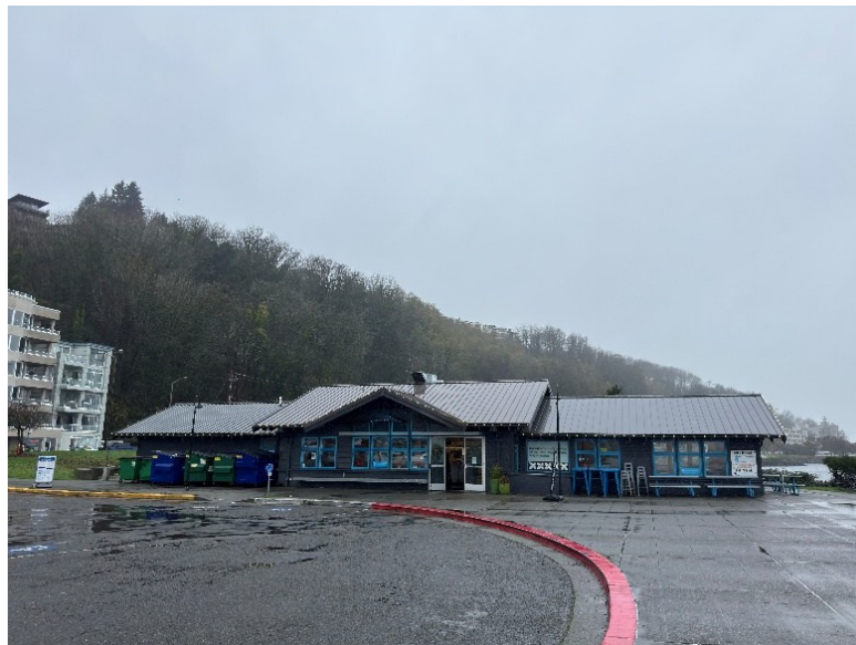
Figure 1 - Exterior Looking North
