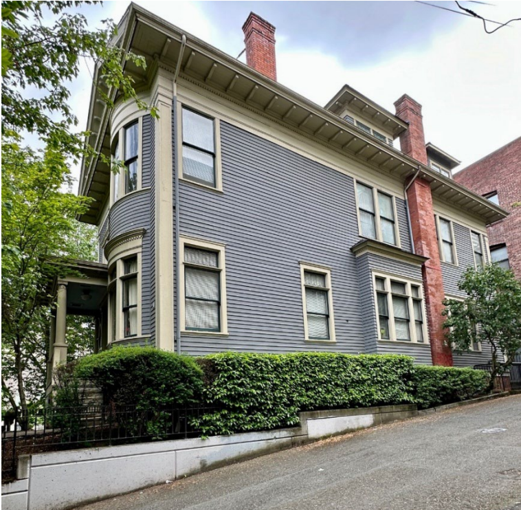
Figure 17: Northwest corner of building, at alley.
