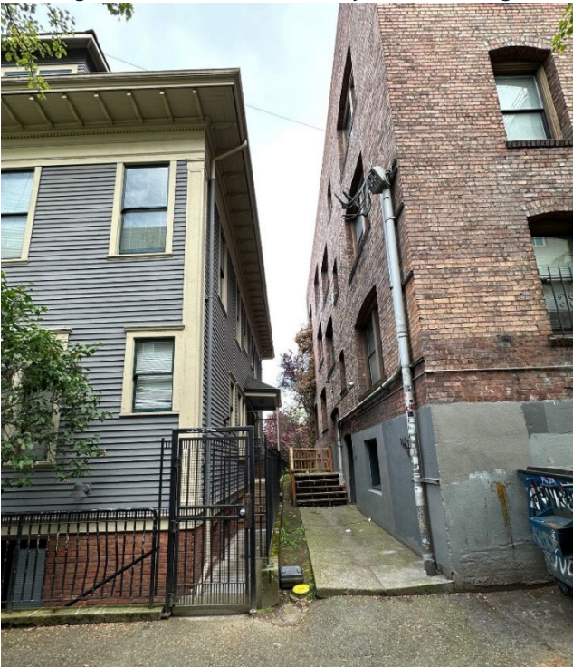
Figure 19: Rear of Phillips house, showing proximity to Maximillian Apartments.
