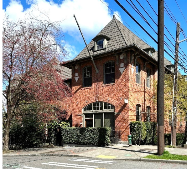
Figure 5 : Old Fire Station #25 1406 Harvard Ave Sommerville & Cote, architects
