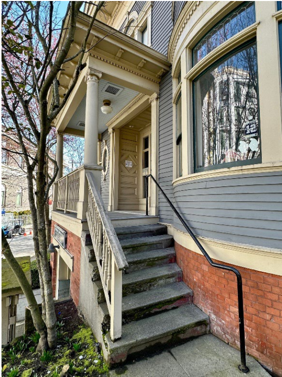
Figure 12: Stairs to entry porches.
