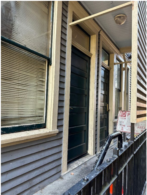
Figure 22: Rear apartment doorways.
