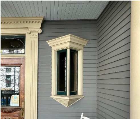
Figure 15: Oriel window at 713 E Union St.
