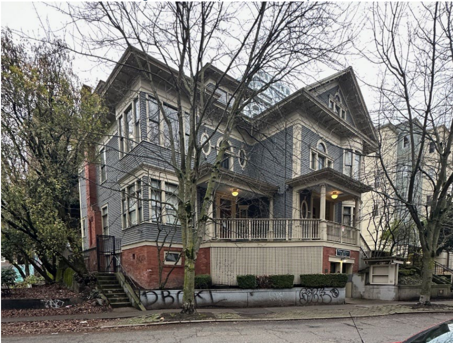
Figure 23: Northeast corner of Phillips house.
