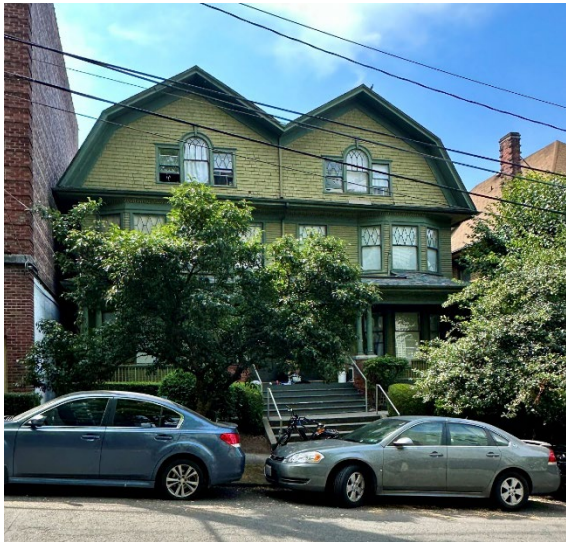
Figure 4 : “Double house” at 1411 Boylston Ave Josehans and Allen, architects
