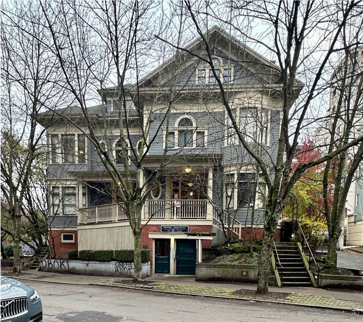
Figure 1: Phillips house, north facing primary elevation on E Union St.
