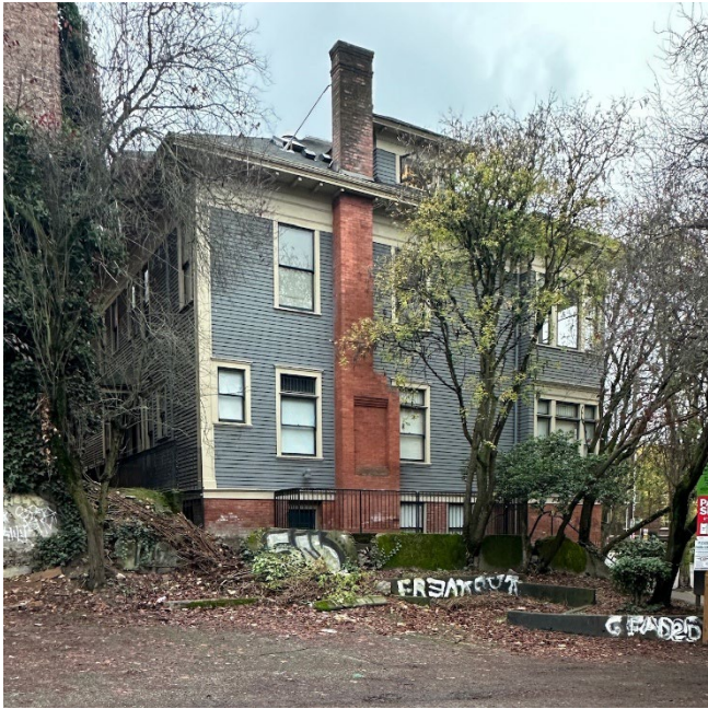
Figure 25: East side of Phillips house from adjacent parking lot.
