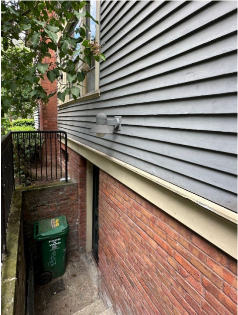
Figure 21: Basement stair on west side of building, along alley.
