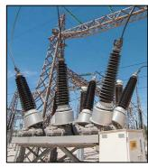
**Circuit Breakers** – A protective device that interrupts electrical current during abnormal conditions such as a short circuit or overload. Protects the transformers and related equipment from damage and prevents widespread outages.
