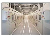
**Switchgear** – Electrical disconnect switches, fuses or circuit breakers used to control, protect, and isolate electrical equipment. Also used to de-energize equipment to allow work and clear short circuits.
