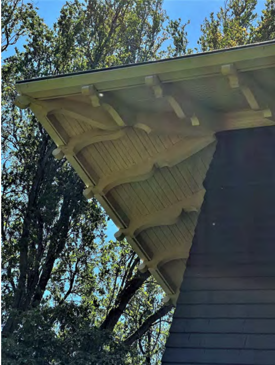
Figure 19. Large, intricately carved rafter tails support the roof, including the roofs over the dormers, front porch, and rear porch. (Author photo)
