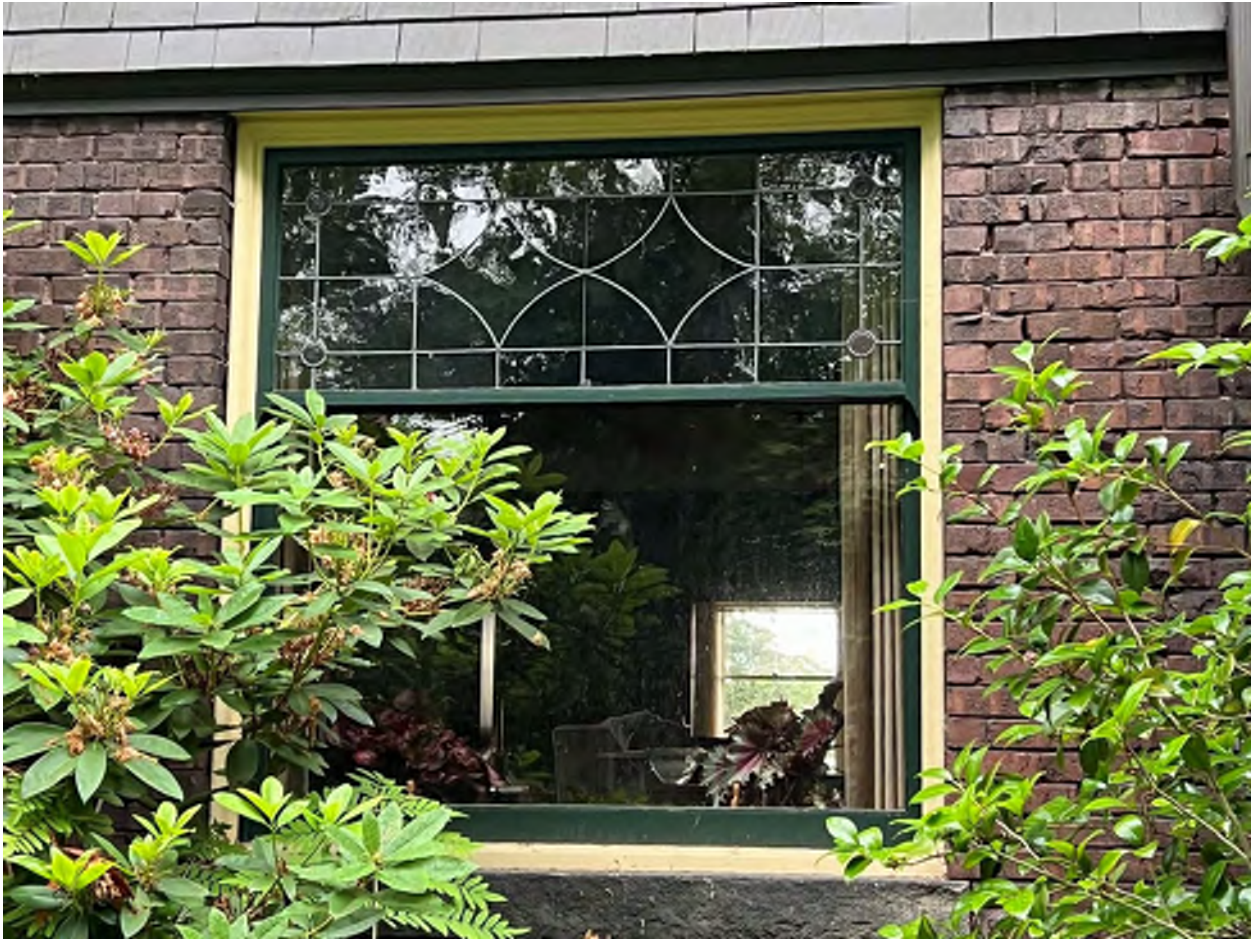
Figure 21. Double hung window with leaded glass in the upper pane. This window type, with two curved diamonds in the center, appears on the first floor. (Author photo)
