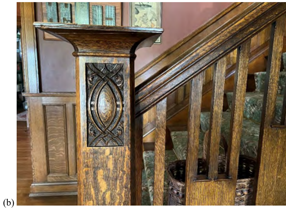
Figure 28. Main stairs. (a) Oak stairway is on the north side of the entry hall. (b) Detail, showing newel post carving and flat three-pronged craftsman balusters, which repeat up the stairs. (Author photos)
