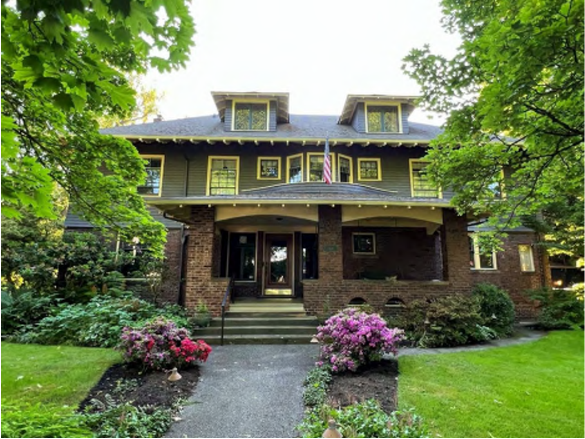
Figure 13. The front (eastern) elevation of the Burwell House appears largely unchanged by time. (Author photo)
