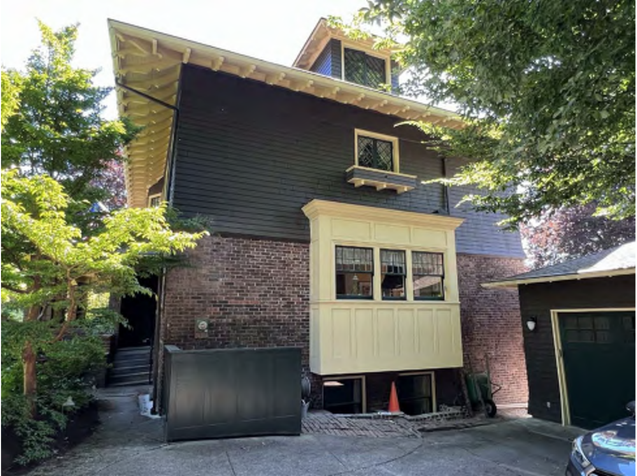
Figure 26. The north elevation of the Burwell House. (Author photo)
