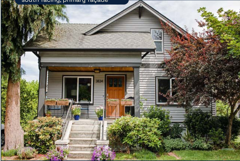
south facing, primary façade
