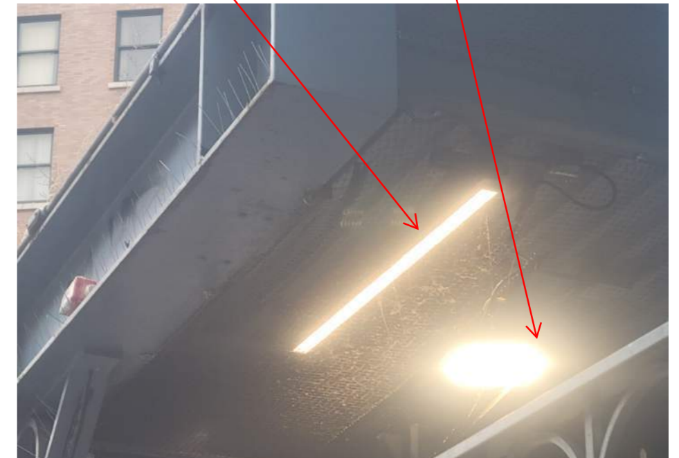
Light fixture at the 3rd Avenue Entrance.
