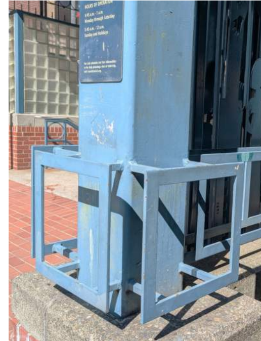
Existing "Pioneer Blue" Paint Color (Exterior) New work to be painted to match
