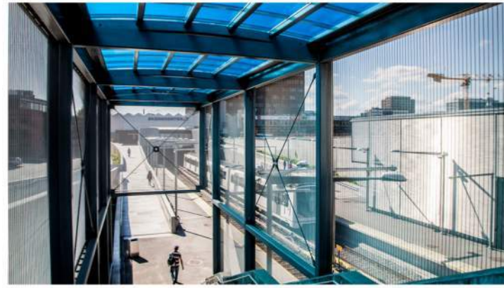
METAL SCRIM PROJECT EXAMPLE Transparency of scrim allows for highlighting the station structure
