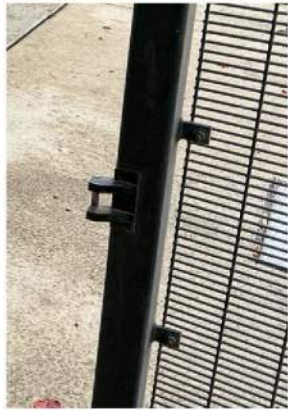
CLIP EXAMPLE Clip attachment
