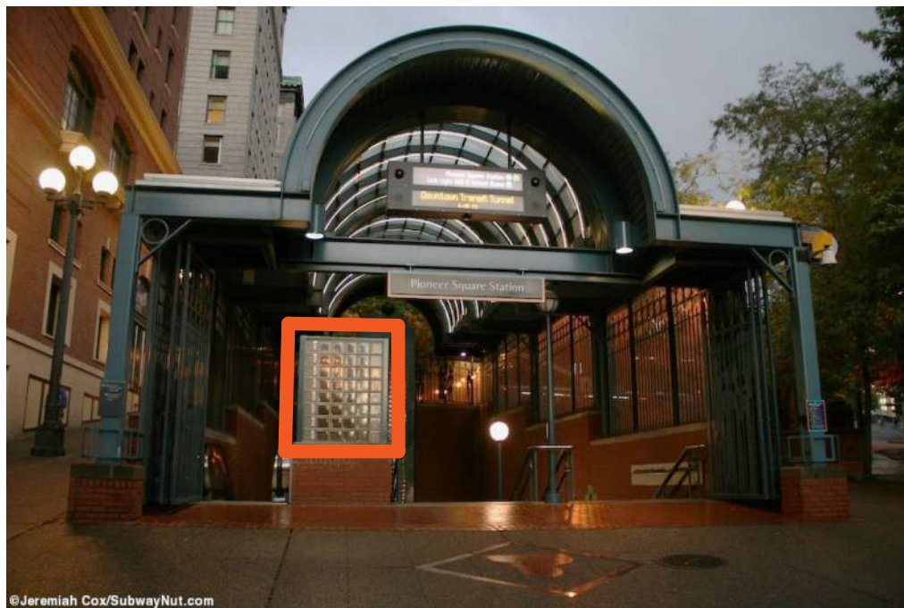
EXISTING PLINTH COVER
