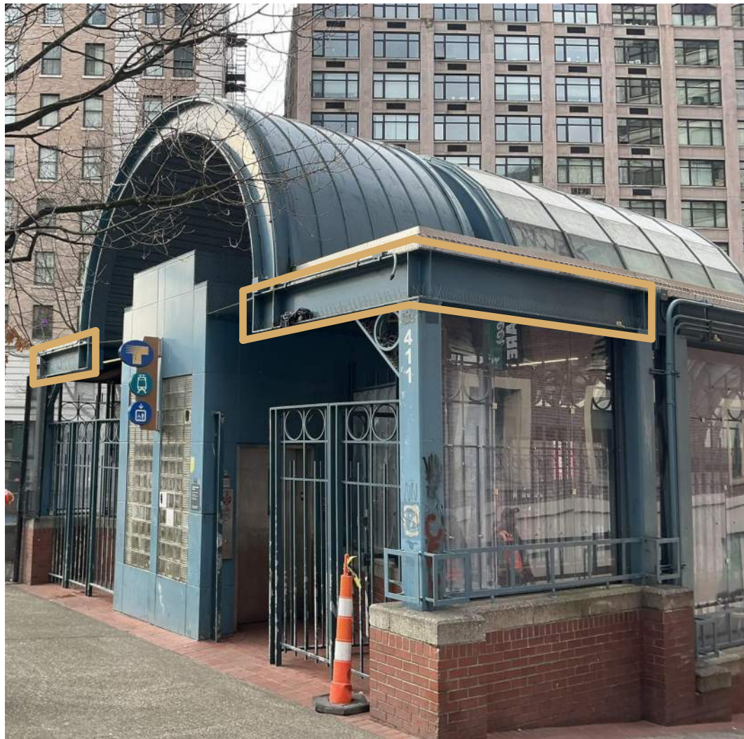
EXISTING FACADE - 3RD AVE / ELEV ENTRY
