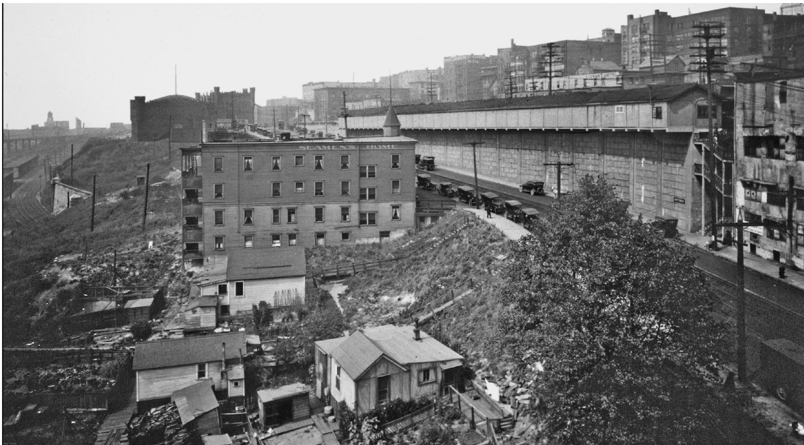
circa 1915- widening of market arcade over new concrete retaining wall on Western Avenue
