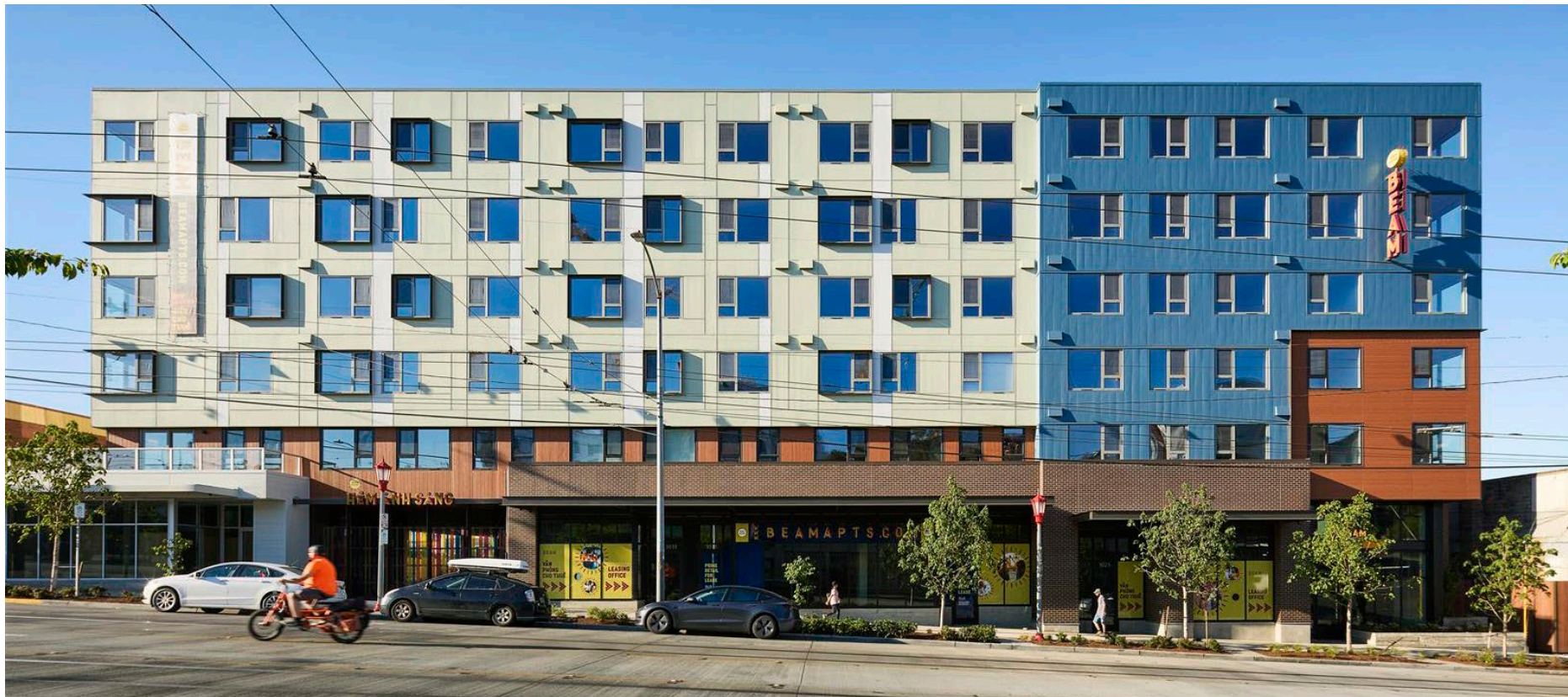
BEAM Apartments - Brick podium with canopies that emphasizes the retail base. © Tiscareno Associates
