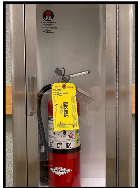
Fire extinguishers must be annually inspected and serviced
